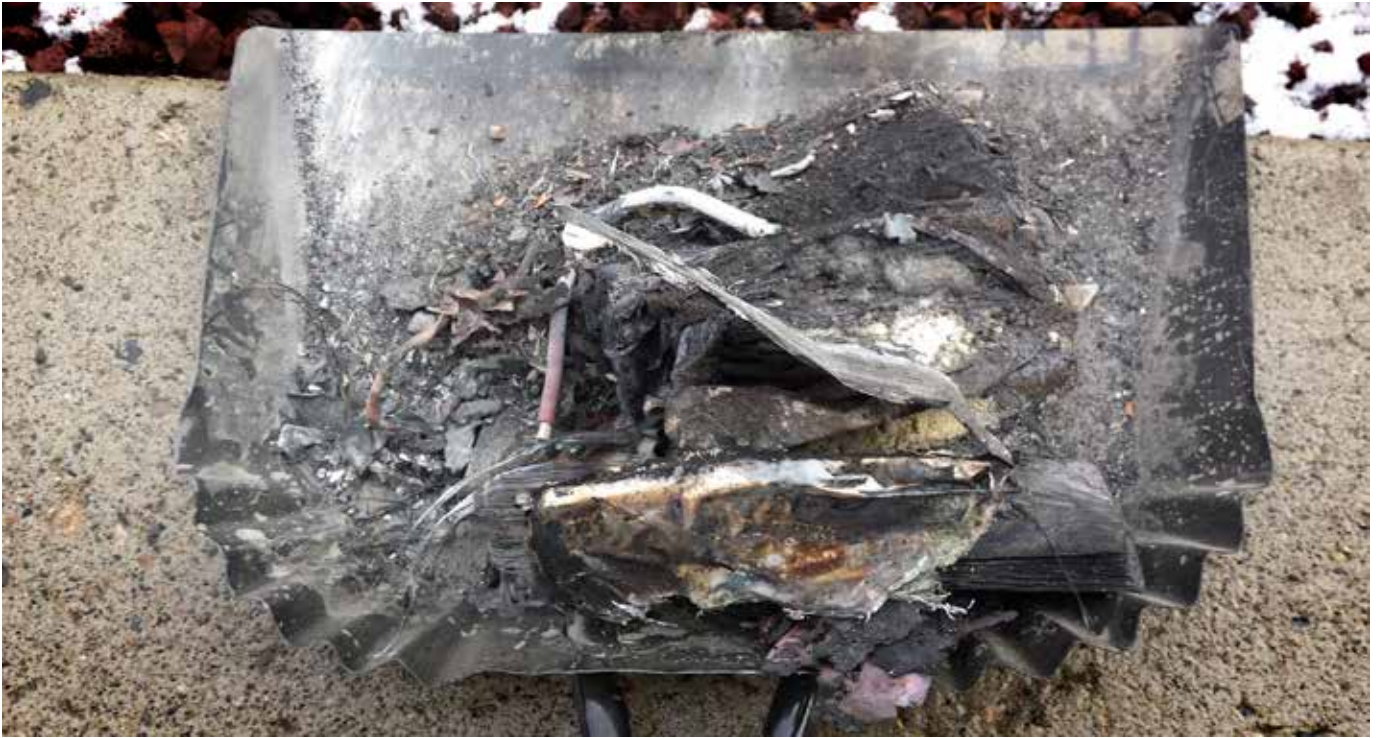
This is a 5S 3300 mAh lipo battery pack that failed while it was being charged. Fortunately this one was caught before it caused any major damage to the house.
