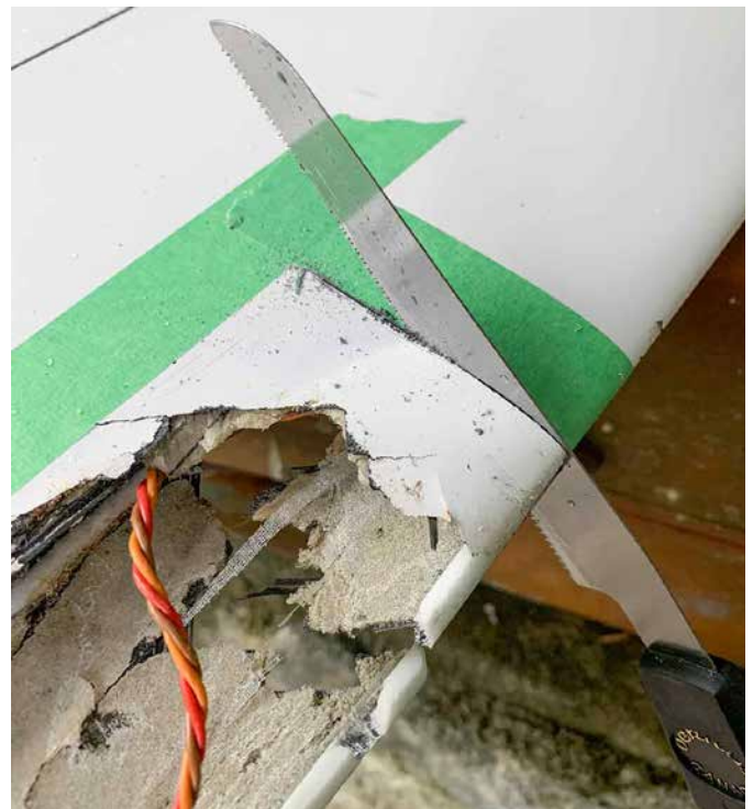
Cutting out the destroyed sections, right back to the spar.
